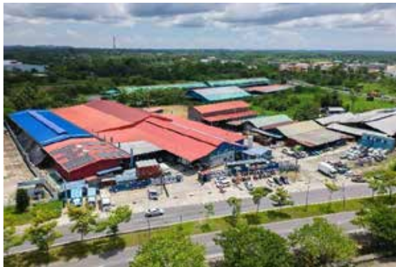
Sandakan Sibuga Plant 1
